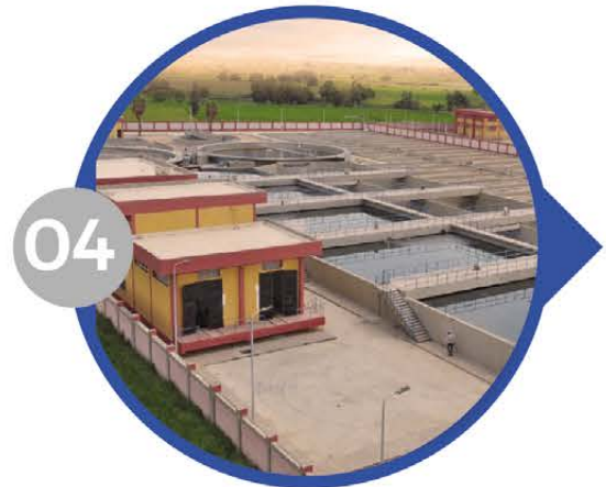
WATER & WASTEWATER TREATMENT PLANTS
